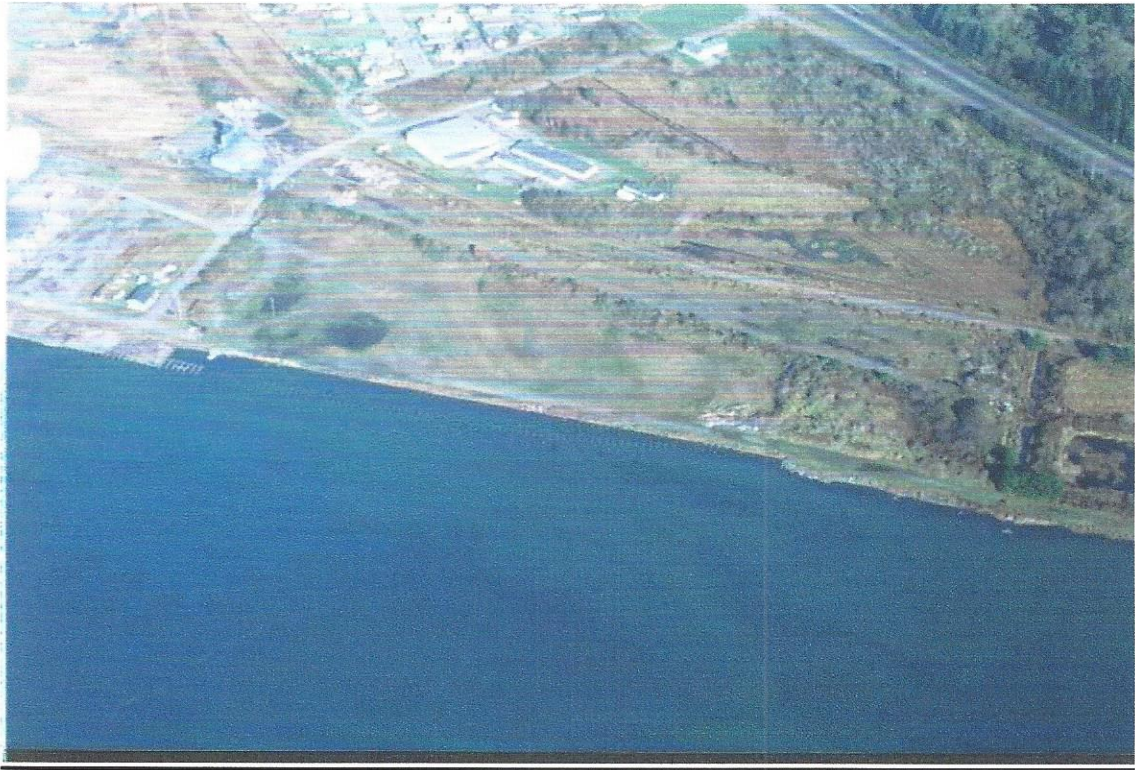
Fields Landing Site
